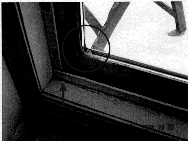
Photo 5: Window Wood Damage and Seal Failure.
