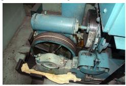
Elevator replacement in similar buildings has been running in the order of **\$175,000** or more and replacement is projected for **year 8**. It should be noted that because of code requirements it is nearly impossible to do partial updates to the elevators without close to complete replacement, but replacement of parts is fine. If parts can be sourced and service is satisfactory, continue to defer replacement.
