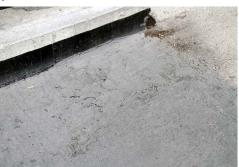
No signs of current leakage were noted on the underside of the slab and with maintenance, the surface should last another **11 years** on a revised **25 year cycle**. Current dollar cost to put a top lift on the pavement should be about **\$22,000**.
