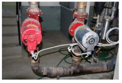
A fractional-horsepower Taco 006-BCF-IFC pump has been employed to circulate domestic hot water to the apartments. These have a typical life expectancy of around **9 years**, but can be run to failure with no real problem for the building. Allocate **\$1,050** for an equivalent pump in **year 5**.
