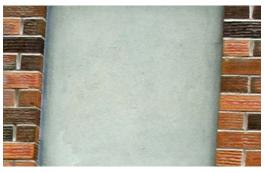
In the order of **15,000 sq ft** of brick veneer, worth in the order of **\$337,500** in current dollars, has been used as the main exterior cladding on the building. Some brick was replaced and general repairs done in 2007. It is the opinion of the author of this report that the brick has the potential to have an indefinite service life if it is adequately maintained over the coming years.
