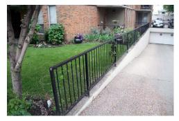
In 2000 about **220 ft** of factory finished fencing was added to the east and west boundaries of the site (the "High Steel Fence"). It will require painting and repairs over the coming years, but painting may be deferred for a number of years. Allocate **\$2,800** for the maintenance of the east and west fence on an **8 year** cycle starting in **year 9**.
