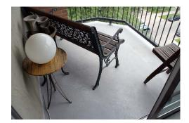
The balcony decks appear to be un-coated concrete. It is recommended that the group consider having a pedestrian-grade urethane coating (or equivalent) applied to extend the life of the concrete. As this would be an improvement, no funding has been shown in the reserve study.
