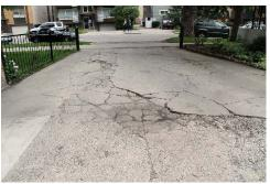
Replacement concrete flatwork has currently been estimated to have a service life of from 20 years to life of the project. Allocate funding for 15% replacement of the new concrete in year 21 and every  $8^{th}$  year subsequent.
